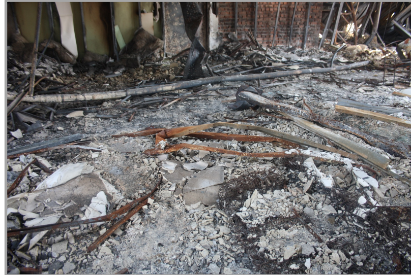
"Epicentr" shopping center, Chernihiv after a fire caused by projectiles. Remains of unburned materials. Burnt machinery
